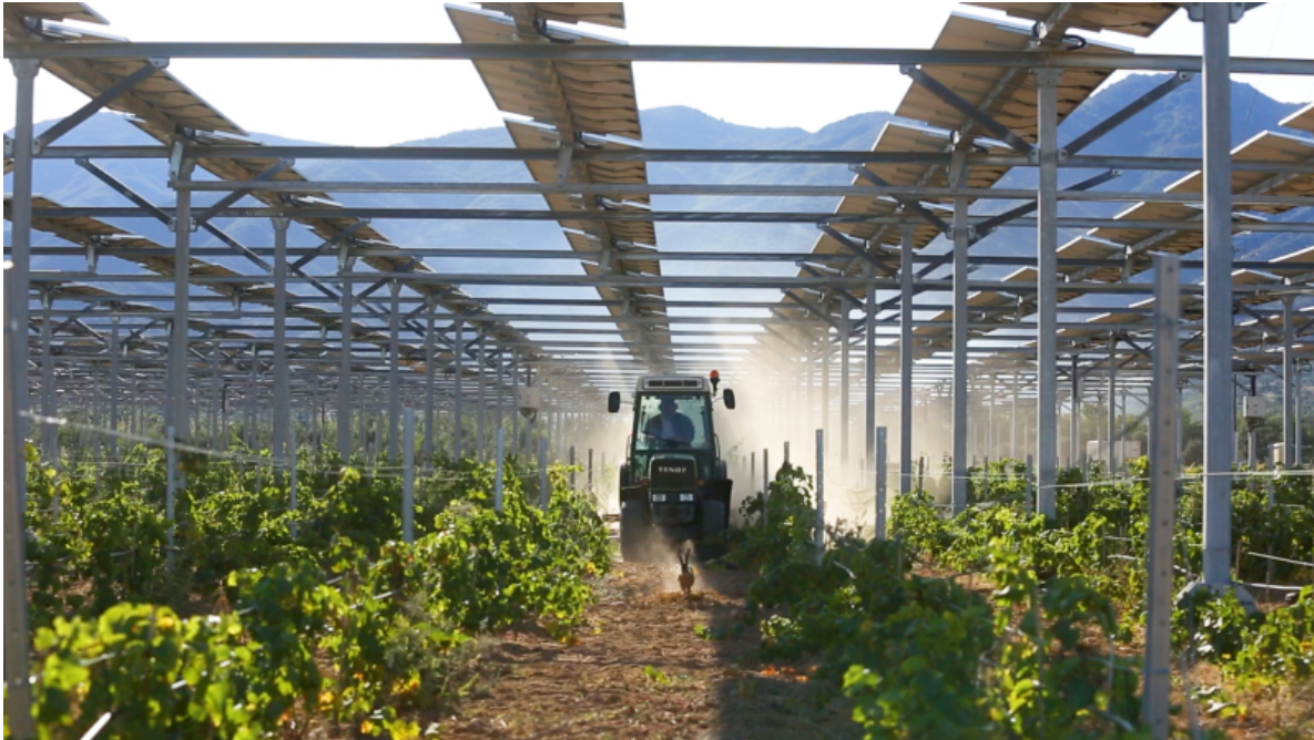
Figure 18. An agrivoltaic system in France produces power and creates a high level of control over insolation, humidity, and protection from wind and pests. ( Sun'Agri 2020)
