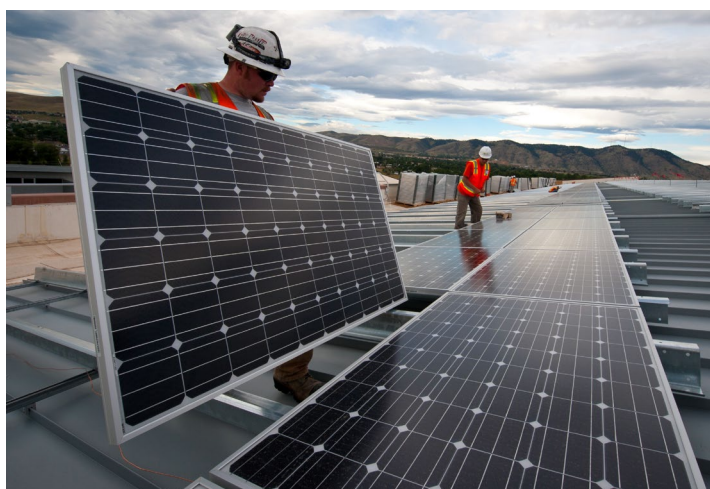
Figure 13. Workers install monocrystalline solar panels on a commercial rooftop. (U.S. Department of Energy)
