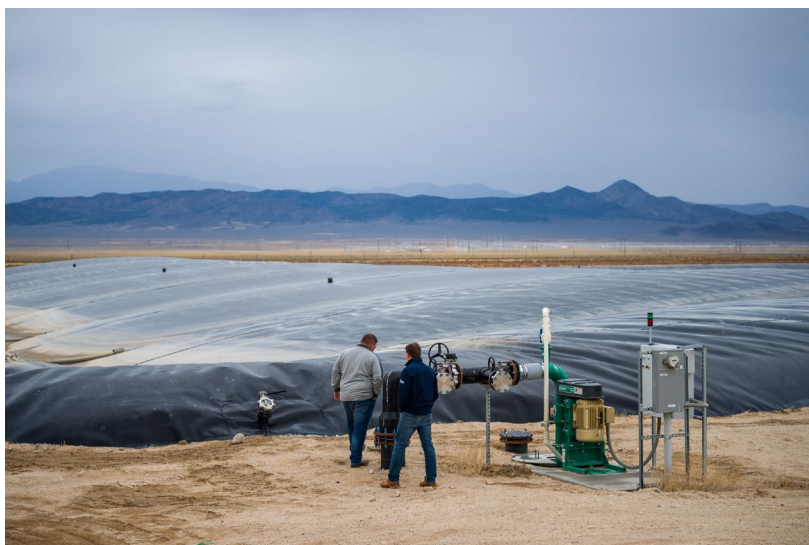
Figure 23. A biogas digester produces methane at a hog farm in Milford, Utah. (Trent Nelson of the Salt Lake Tribune)
