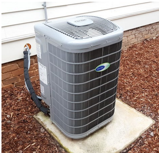
Figure 24. An air source heat pump provides heating and cooling more efficiently than a furnace and air conditioner. ( Brecha 2021)
